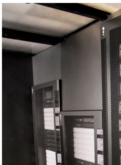
Blanking space from different height racks.
